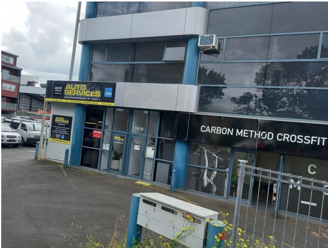
Image 1: Auto services and Carbon Method Crossfit are some of the tenants
