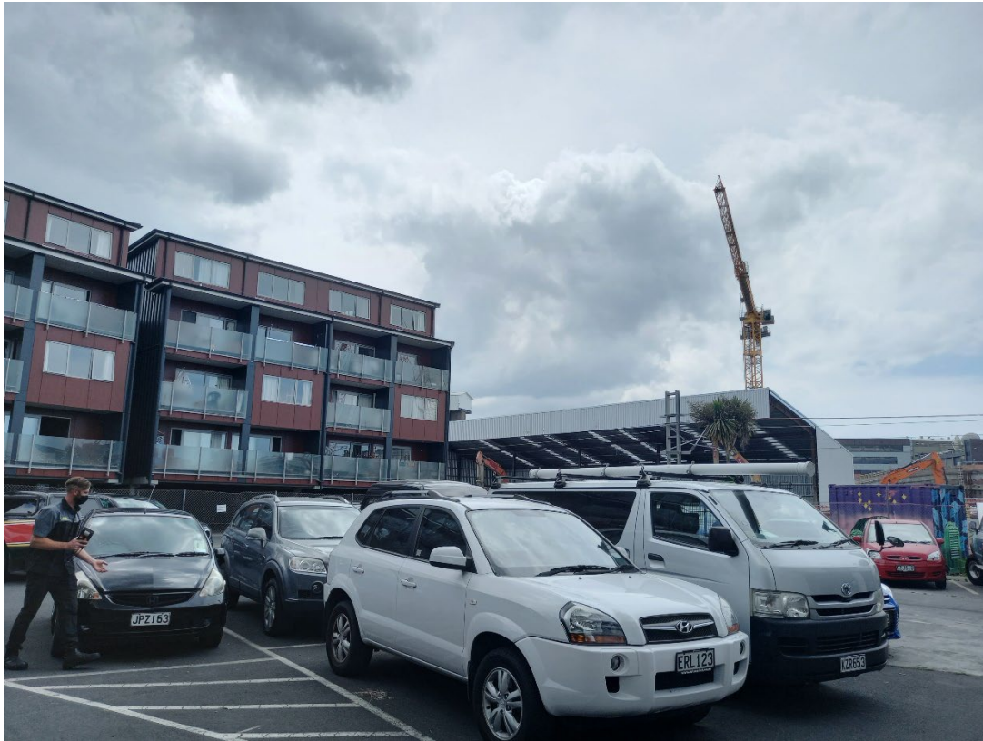
Image 3: Apartment building adjoining the site
